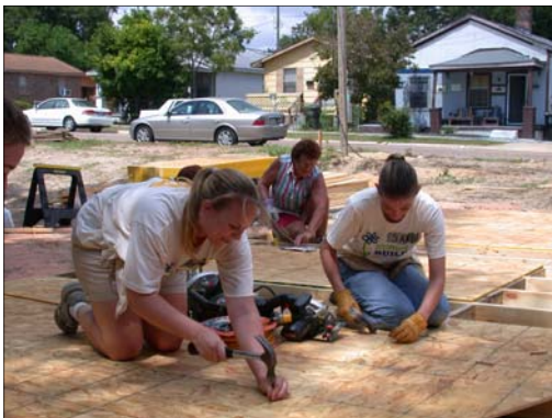
Jeanie and Sara secure the OSB to the walls.
