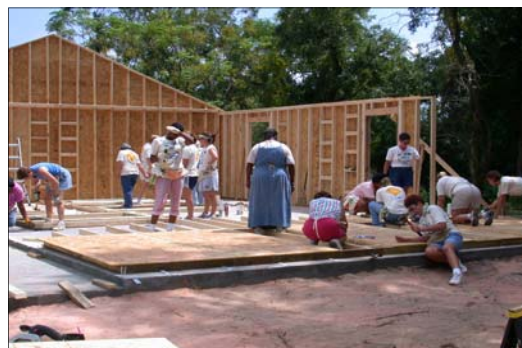
Jeanie and Sara secure the OSB to the walls.
